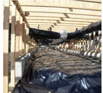
Underfloor Ductwork
