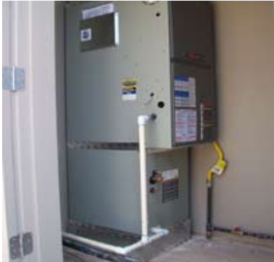
Trane High Efficiency Gas Furnace
